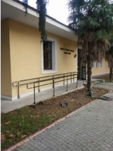
3. Disabled Ramp and Handrail (Gebze Technical University, Turkey)
