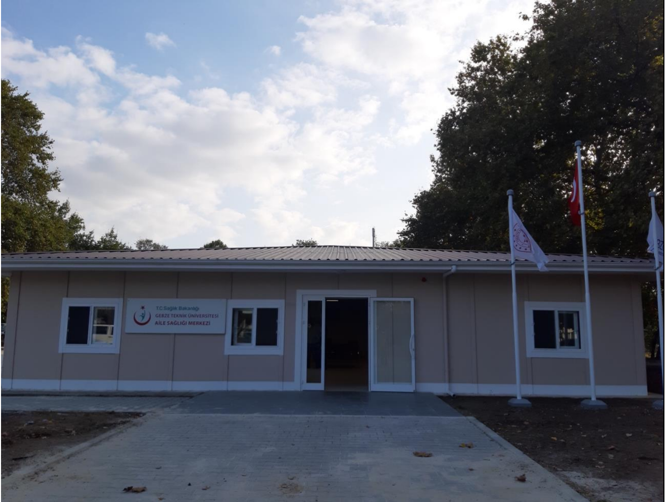
Health center building of Gebze Technical University, Türkiye -1
