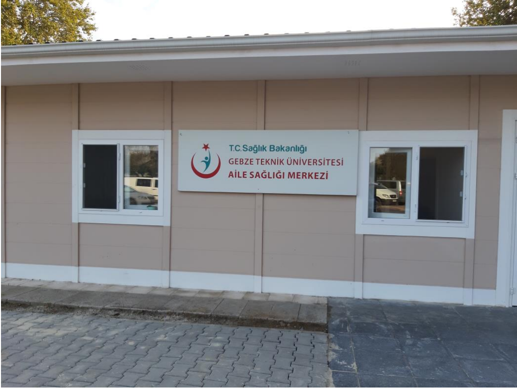
Health center building of Gebze Technical University, Türkiye -2
