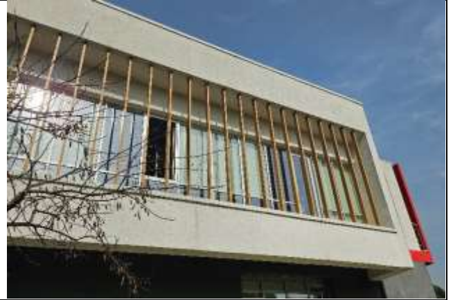
Sun shading elements
