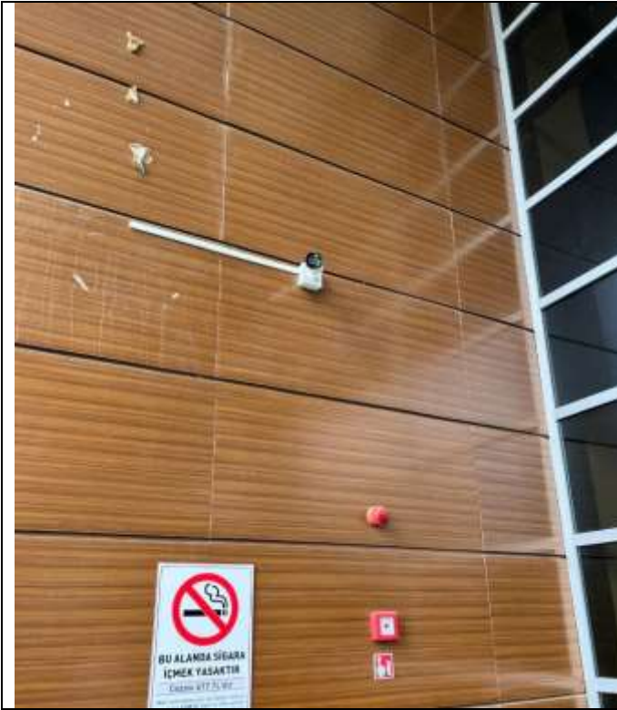
Security and surveillance system
