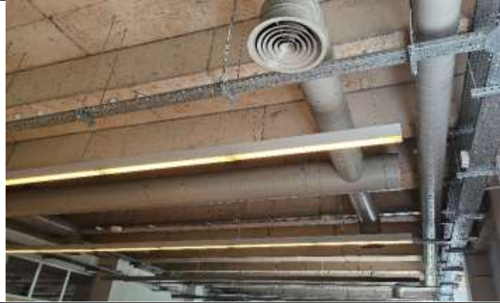
LED lights in the classrooms
