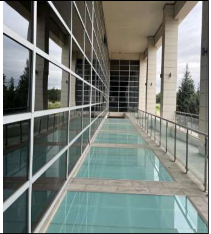
Glass floors providing natural light to basements
