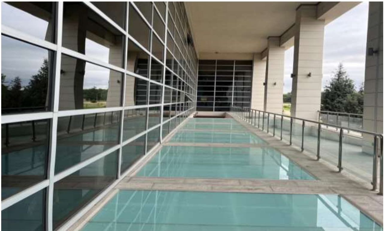
Glass floors providing natural light to basements
