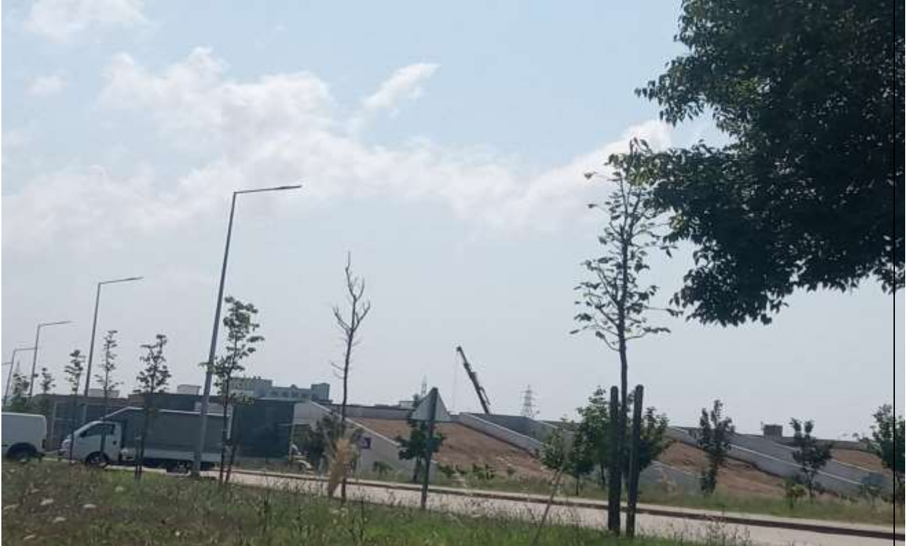
Green roof construction
